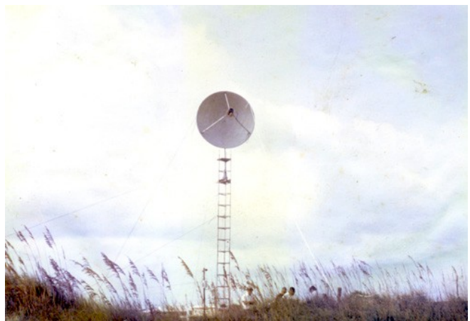
The 6' dish mounted at top of tower, with Rotor. Memory suggests height of tower was about 20'.
