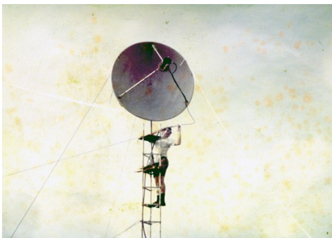
Walt making adjustment to the feed-line dress. Notice the coffee can feed which was popular at the time.
